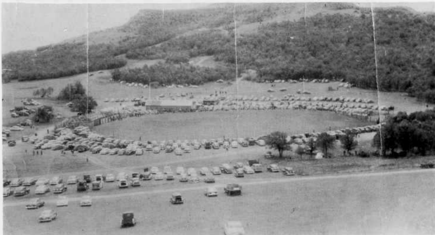
This outstanding photo, probably taken about 1950, shows the rodeo grounds during the event's last years in the Mountains. It is shot from Spectator Hill on the north. The barn, bowery and bar are the buildings on the south side of the arena. Concrete footings for
