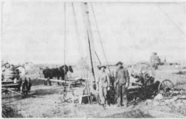
Well drilling at Hazelton
