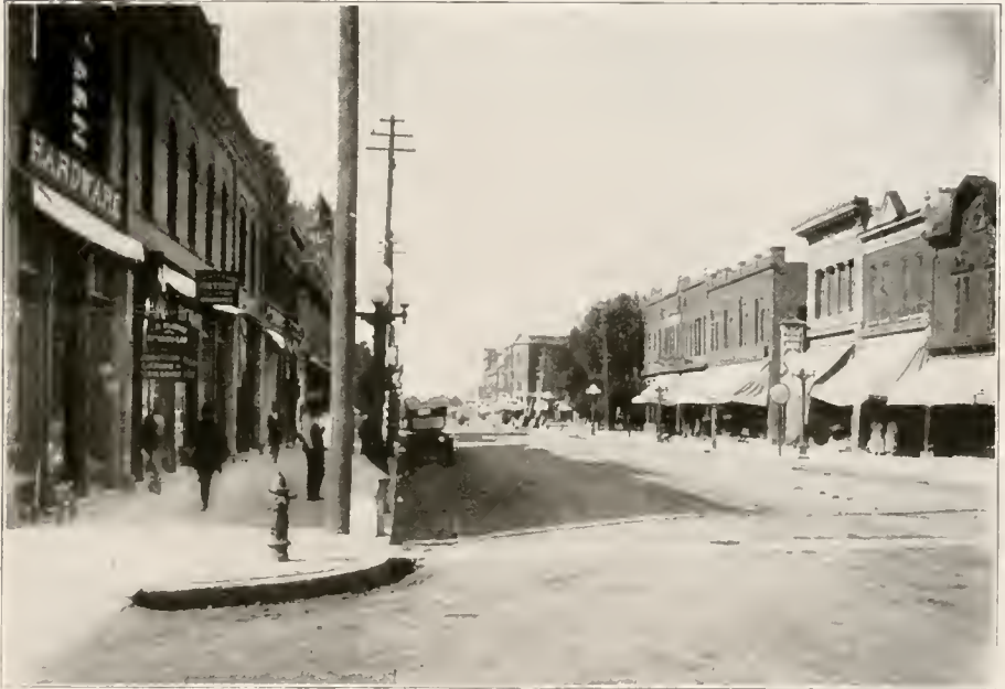
VIEW ON FIFTH AVENUE, JAMESTOWN, LOOKING NORTH
