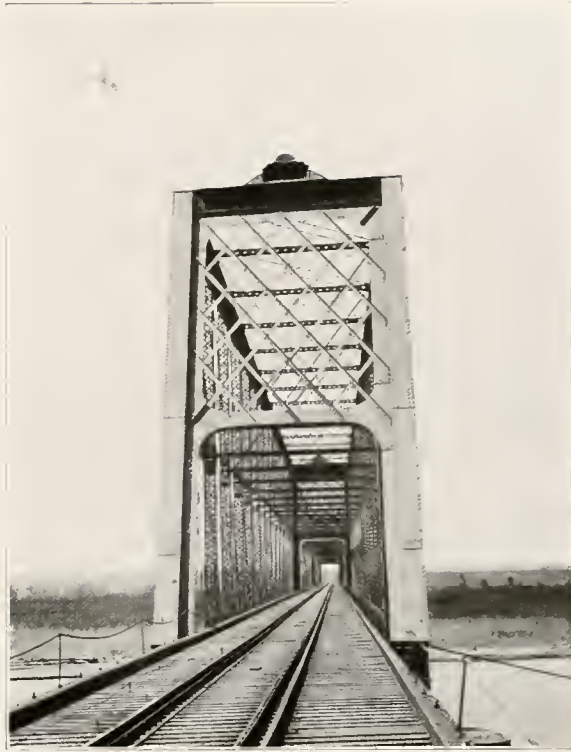
NORTHERN PACIFIC BRIDGE OVER THE MISSOURI RIVER AT BISMARCK
