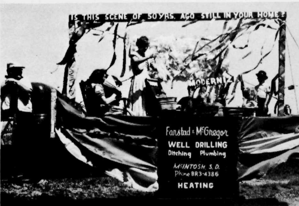
Farstad and McGregor Well Drilling
