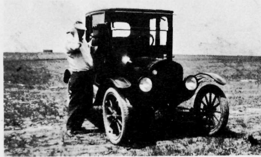
J. B. Smith making the first long distance telephone call. As the telepho ne co. was completing the installation, J. B. drove his car to the edge of town where he made the first telephone call. Year 1924
