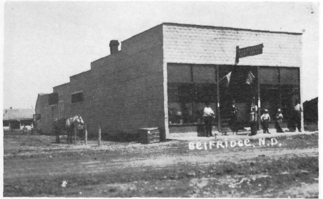
Gas pump installed - sidewalk finished. In the background can be seen Mrs. Smestad and children.
