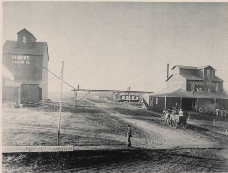
GOOSE RIVER MILLS AND FARMERS ELEVATOR, CITY OF MAYVILLE, TRAILL CO. L. B. GIBBS AND C. S. EDWARDS, PROPRIETORS.
