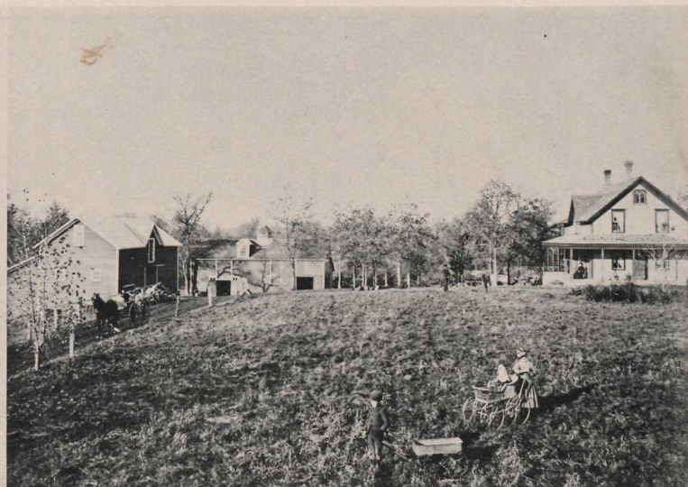
FARM BUILDINGS OF M. J. GUMMER, SEC. 5, MAVVILLE TP., 146-52, TRAILL CO.
