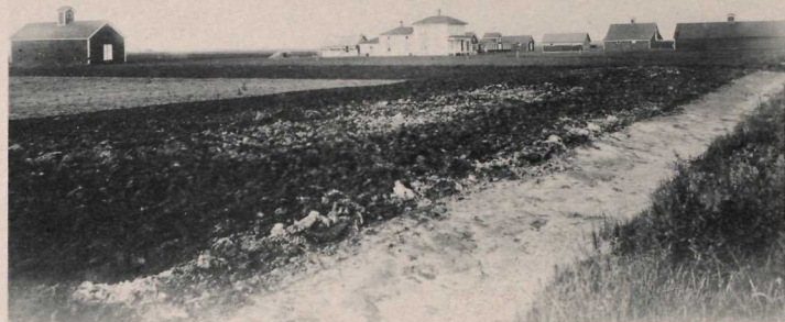
FARM BUILDINGS OF H. D. HURLEY, SEC. 33, CALEDONIA TP. 146 N., RANGE 49 W., TRAIL CO.
