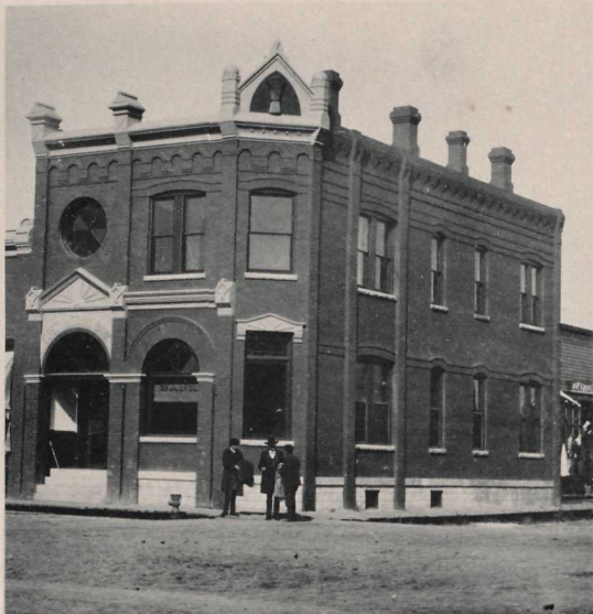
FIRST NATIONAL BANK BUILDING, CITY OF MAYVILLE, TRAILL CO. G. S. ALBEE, Pres't. J. P. HABER, Vice Pres't. J. ROSHOLT, Cashier.
